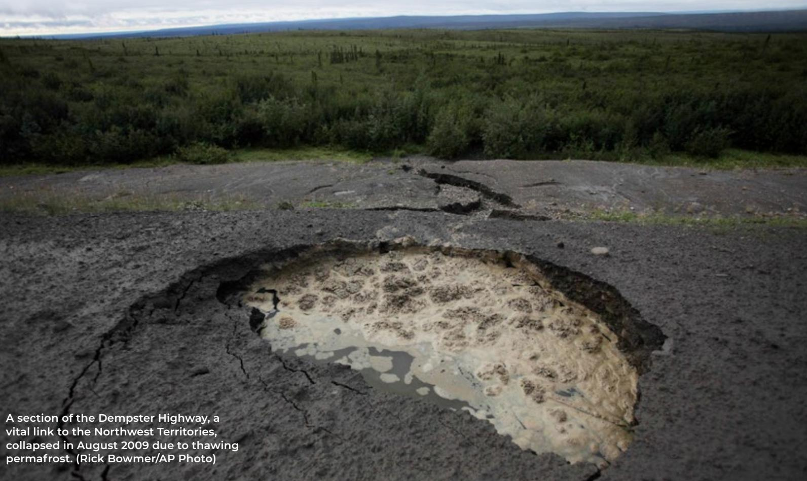
A section of the Dempster Highway, a vital link to the Northwest Territories, collapsed in August 2009 due to thawing permafrost. (Rick Bowmer/AP Photo)
